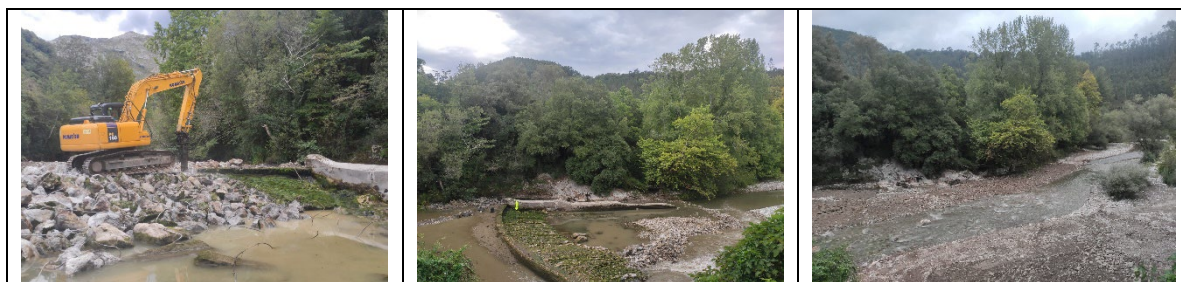
Figure 15. Works on Puentellés dam (sep-2022). River section before and after the dam removal.
