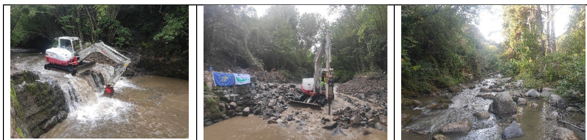
Figure 16. Works on Ferrería de Ojedo dam (sep-2021) and the river section after the dam removal.
