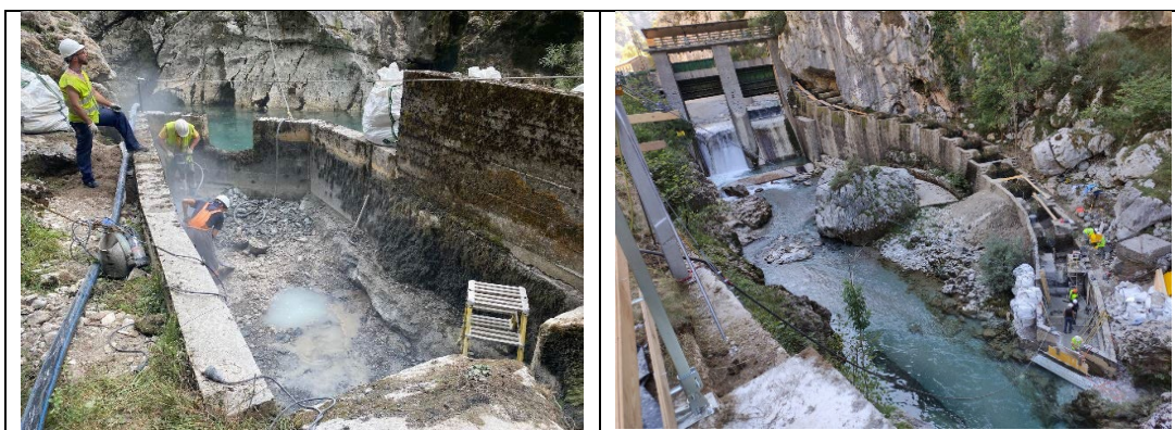
Figure 20. Works on Poncebos fish passage (oct/2022).
