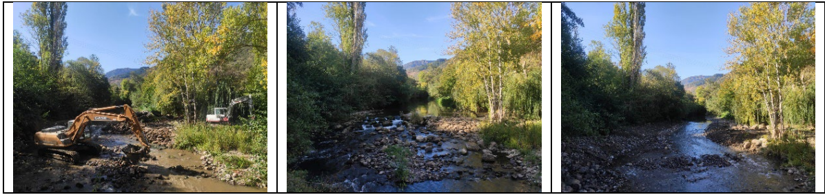
Figure 18. Works on Sotama dam (oct/2023). River section before and after the dam removal.
