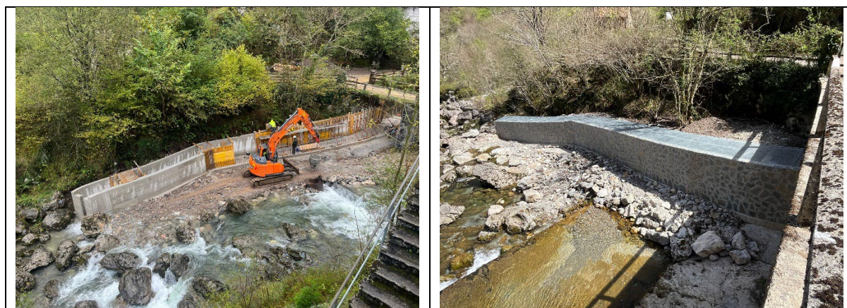
Figure 22. Construction works of Restañó dam fish passage and finished passage (apr-2024).
