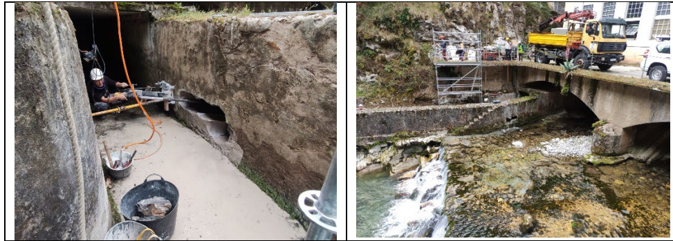
Figure 19. Works on Urdón dam (aug-2022).
